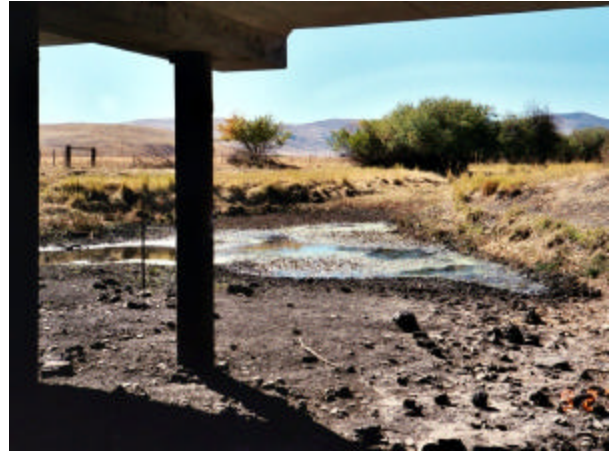
Figure 33. Reach 1 from under Uecker Bridge.
