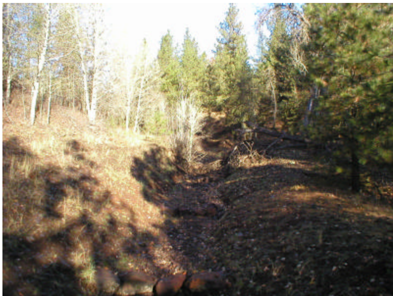
Photo 2. Rock Creek stream channel near Station RC-02, 11/18/04
