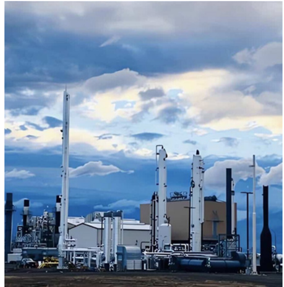
H.W. Hill Landfill Gas Project. Source: Republic Services
